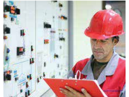
Industrial Panel Rooms
