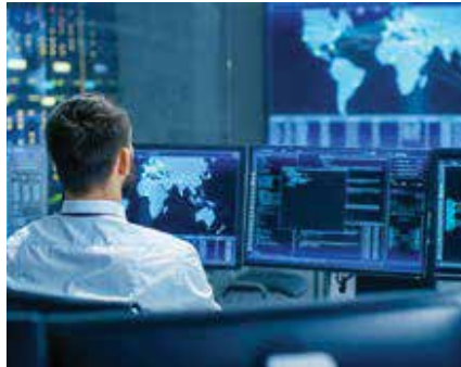
Computer Rooms and Control Rooms
